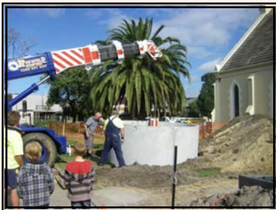
Putting the tank in place
